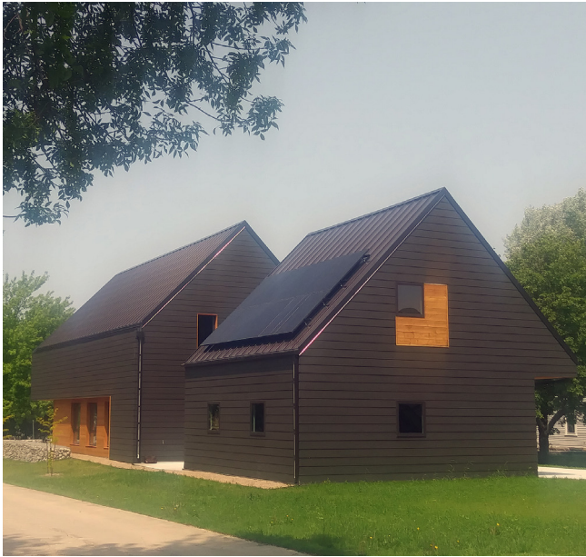
Figure 3. Solar PV installation at PH01:BRK. Photo: Charles MacBride.
